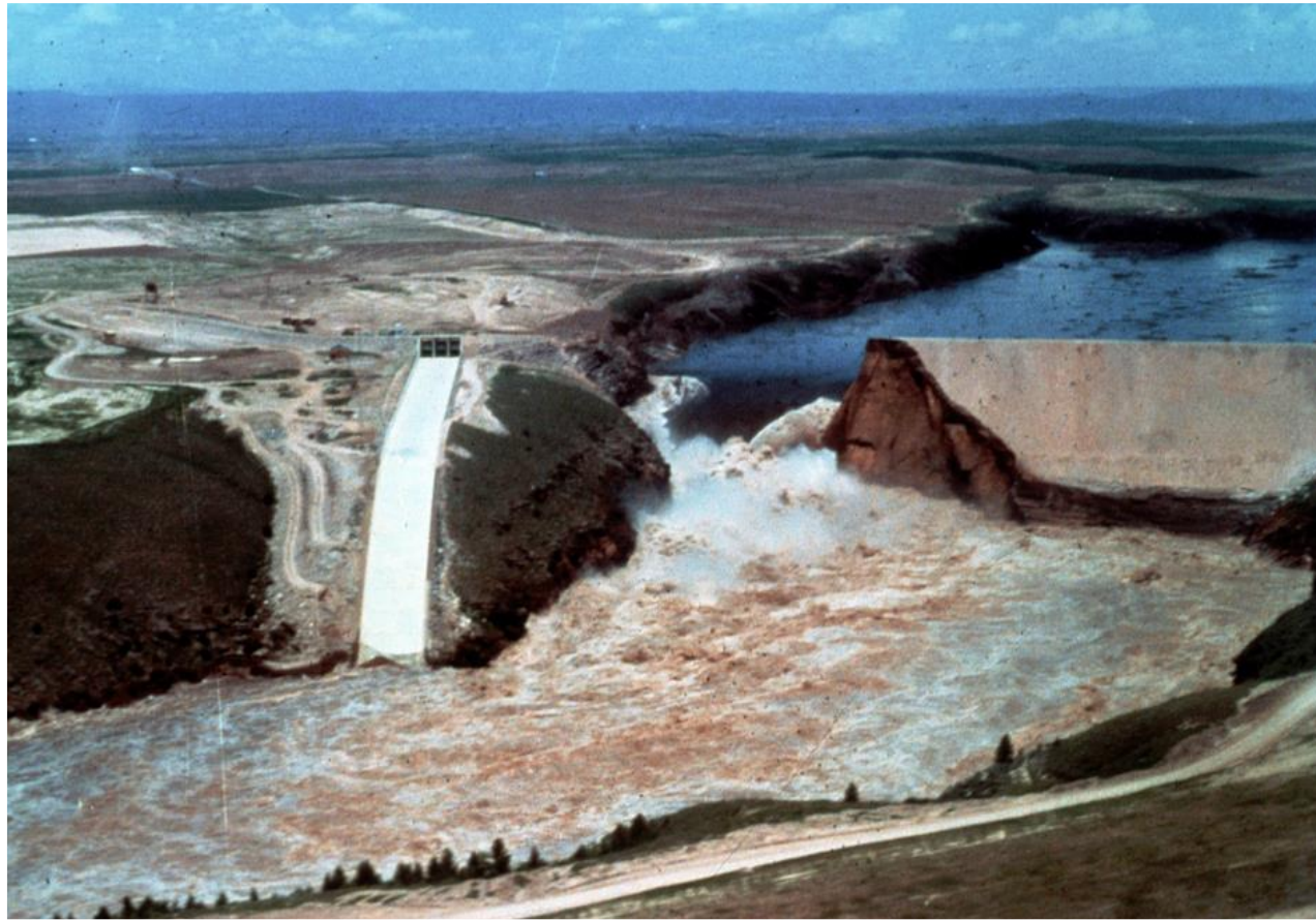
Failure of Teton Dam on June 5, 1976
